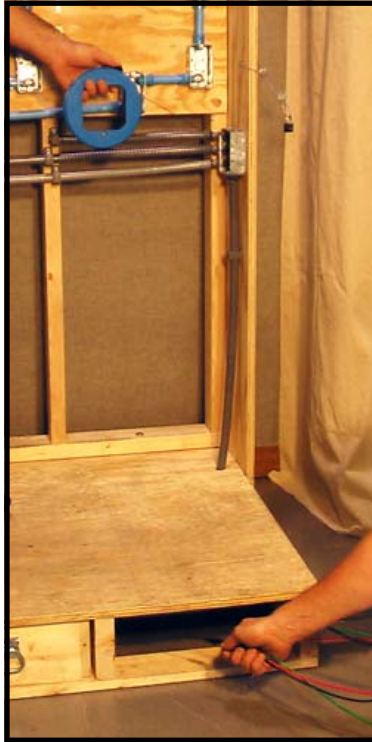
Using Fish Tape to Pull Wires
