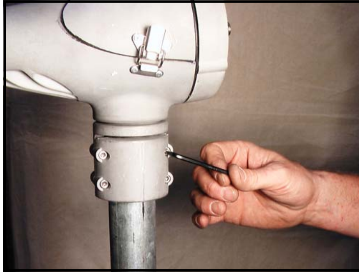
Tightening Mounting Fasteners with Hex Key
