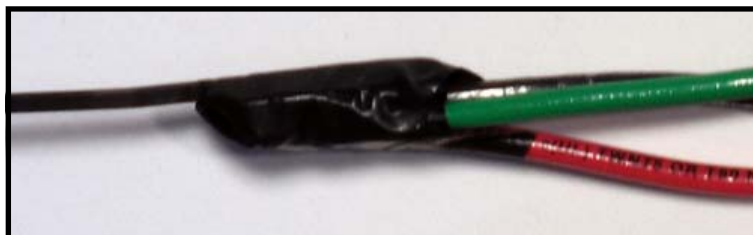
Using Electrical Tape to Splice Wires to Fish Tape
