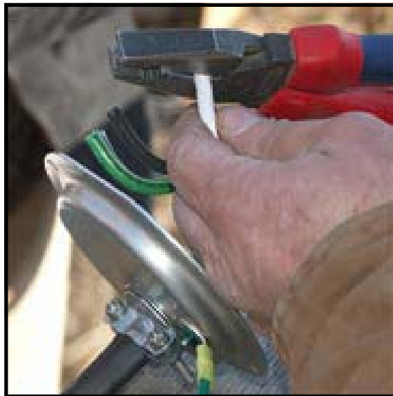
Installing Wind Turbine Wires
