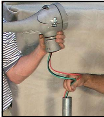
Feeding Yaw Wires into Tower
