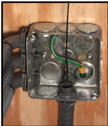
Fish Tape Extending into Junction Box and Out Bottom of Workstation
